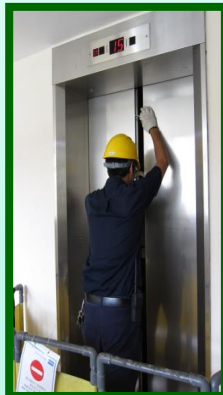
The landing door should be opened not more than a clearance of 90mm in width for checking the position of the lift car
