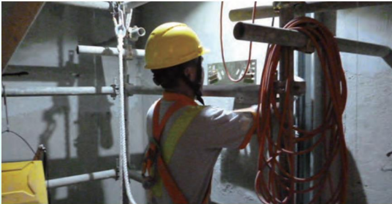
全身式安全帶要掛在升降機槽內的救生繩 Safety harness attached to lifeline inside lift shaft
